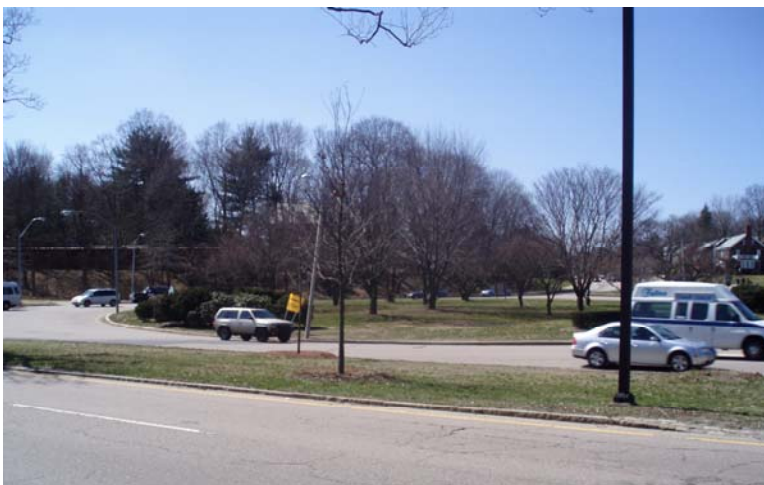
Figure 1.2: Heavy vehicular flows around existing rotaries make merging and navigating dangerous for motorists.
