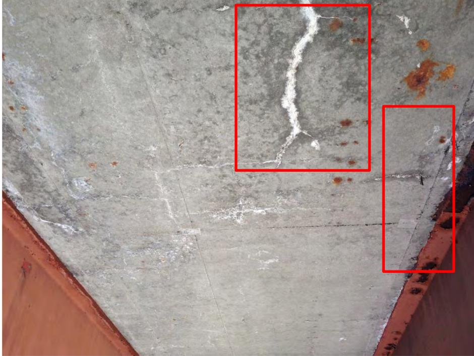
Figure E.7: Cracks and corrosion on the underside of Bridge 4FH, Span 7 deck.
