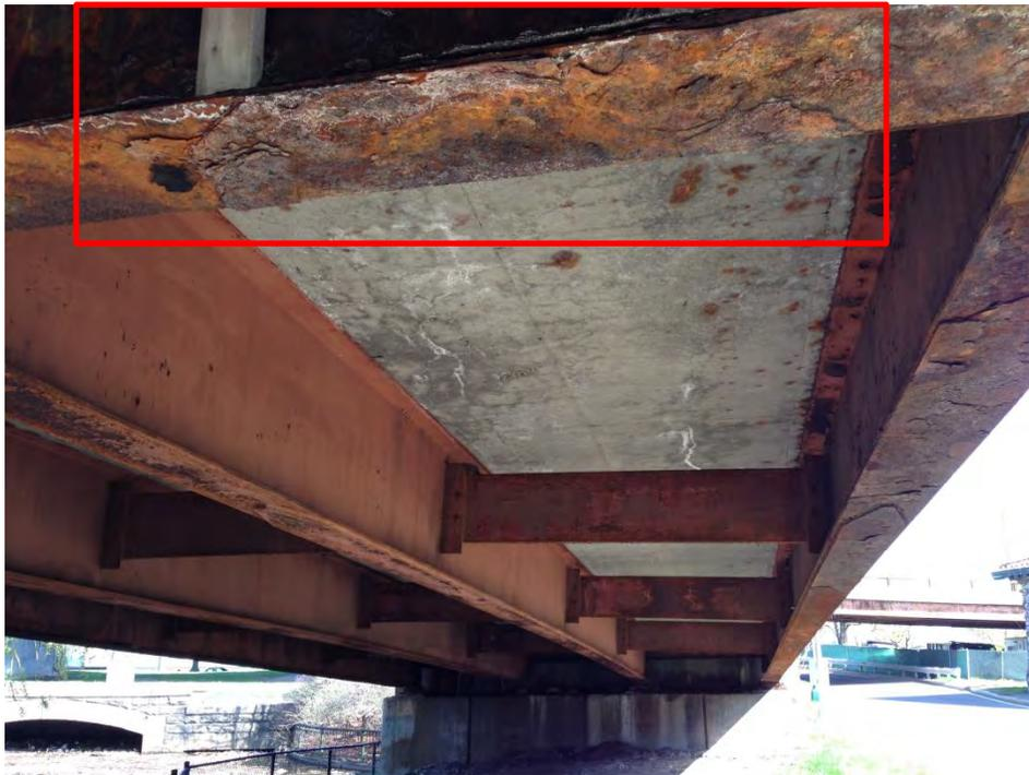
Figure E.2: Underside of Bridge 4FH, Span 7 and delamination on the south end.
