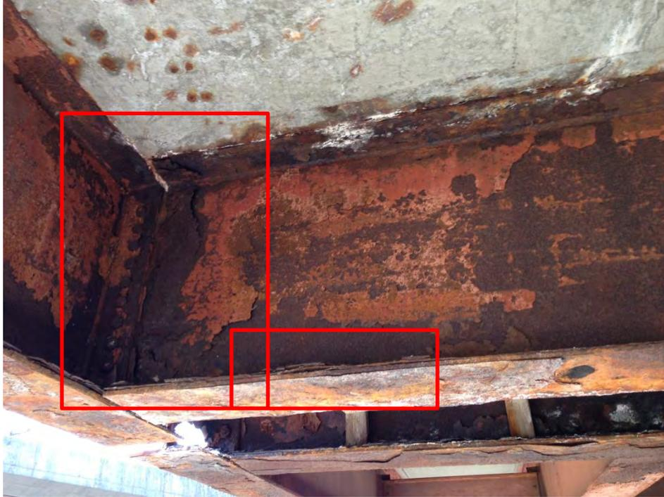
Figure E.5: Corrosion and delamination on the north side of the joint of Bridge 4FH, Span 7.
