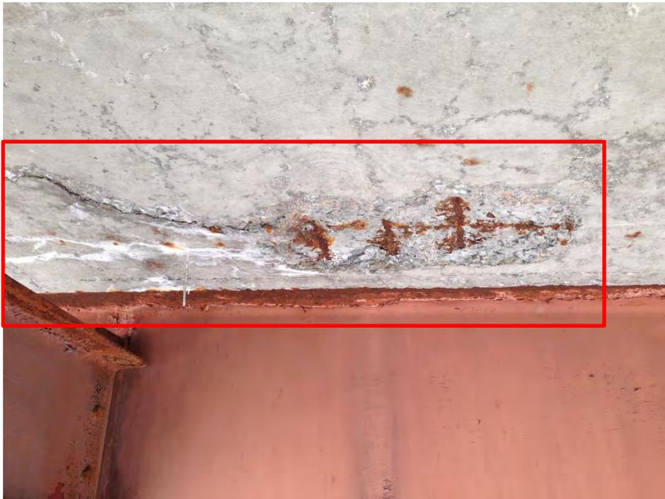
Figure E.8: Concrete spalling and exposed reinforcement on the underside of Bridge 4FH, Span 7 deck.
