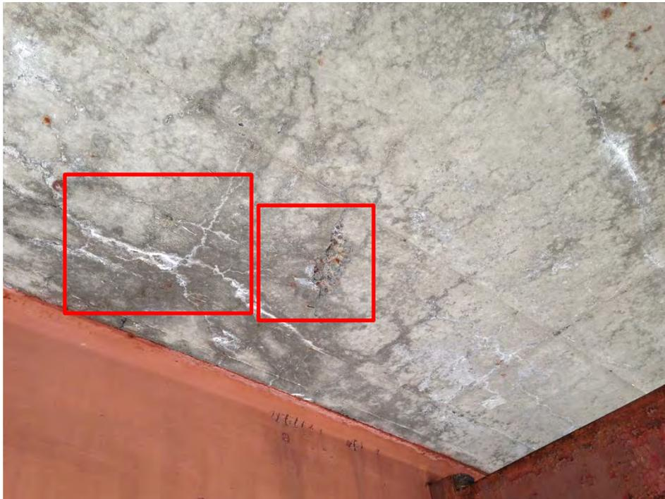
Figure E.6: Concrete spalling and cracking on the underside of Bridge 4FH, Span 7 deck.
