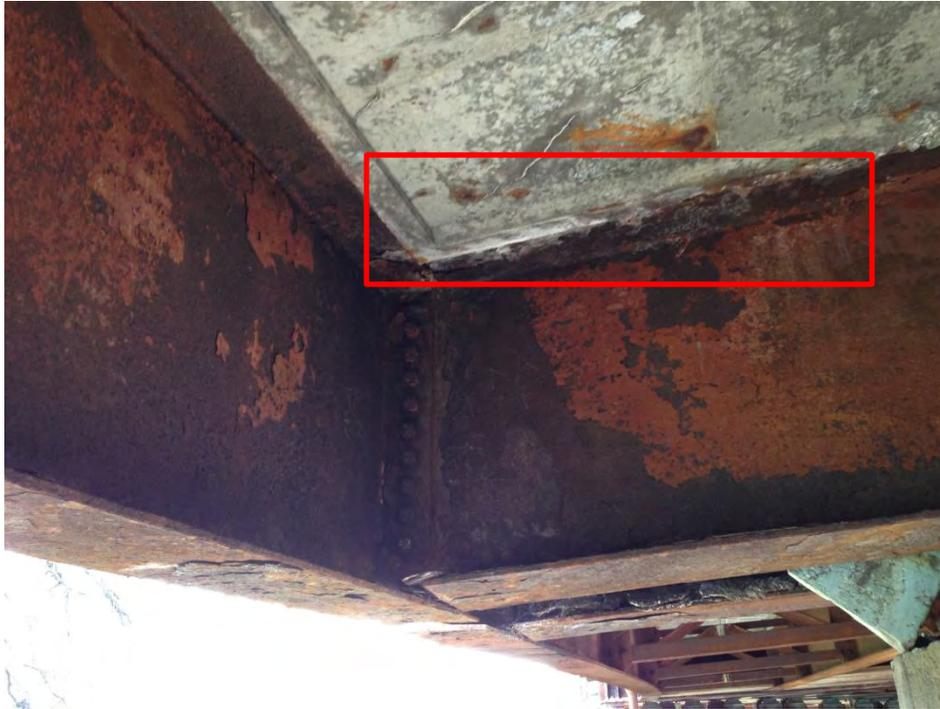
Figure E.12: Corrosion on the north side of the joint of Bridge 4FJ.
