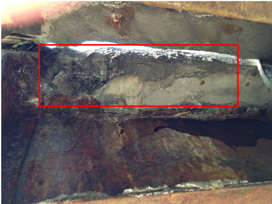
Figure E.11: Concrete spalling under the expansion joint of Bridge 4FJ.
