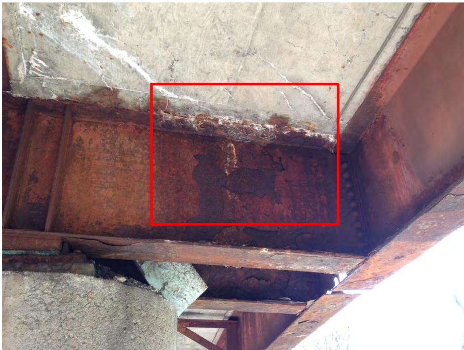
Figure E.13: Corrosion on the south side of the joint of Bridge 4FJ.
