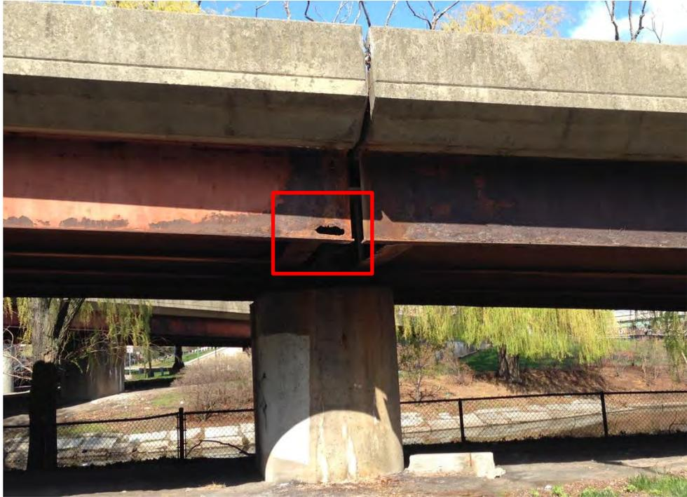
Figure E.3: Section loss on east-side exterior fascia girder on Bridge 4FH, Span 7.
