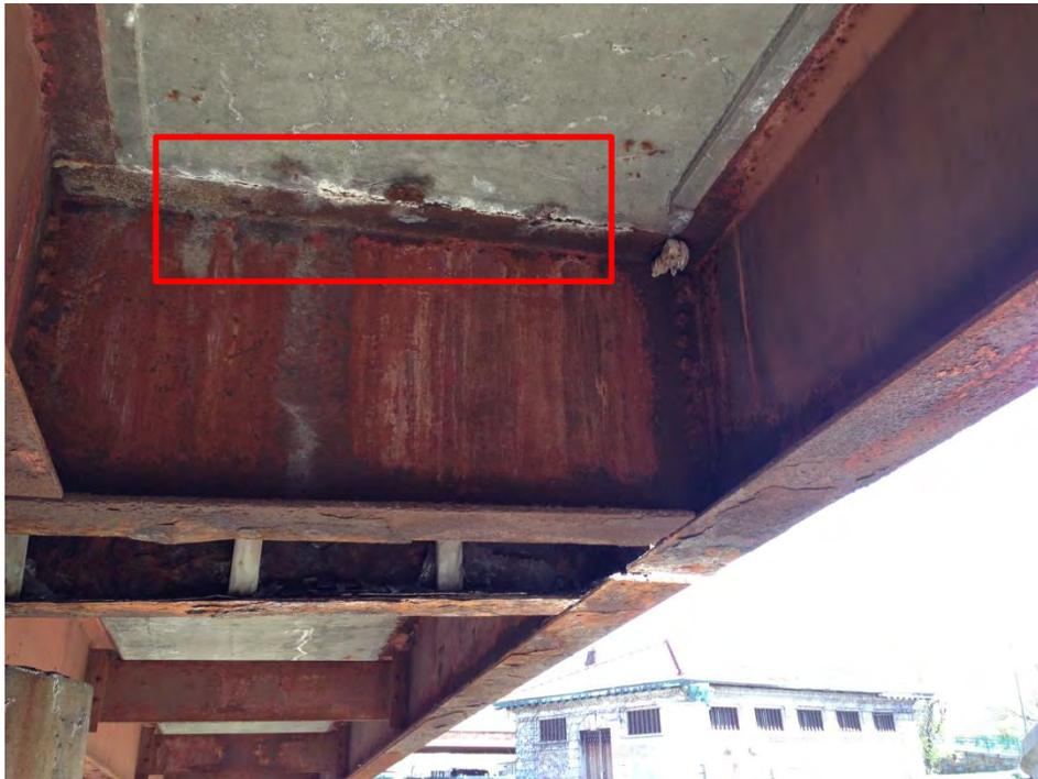
Figure E.4: Corrosion on the south side of the joint of Bridge 4FH, Span 7.
