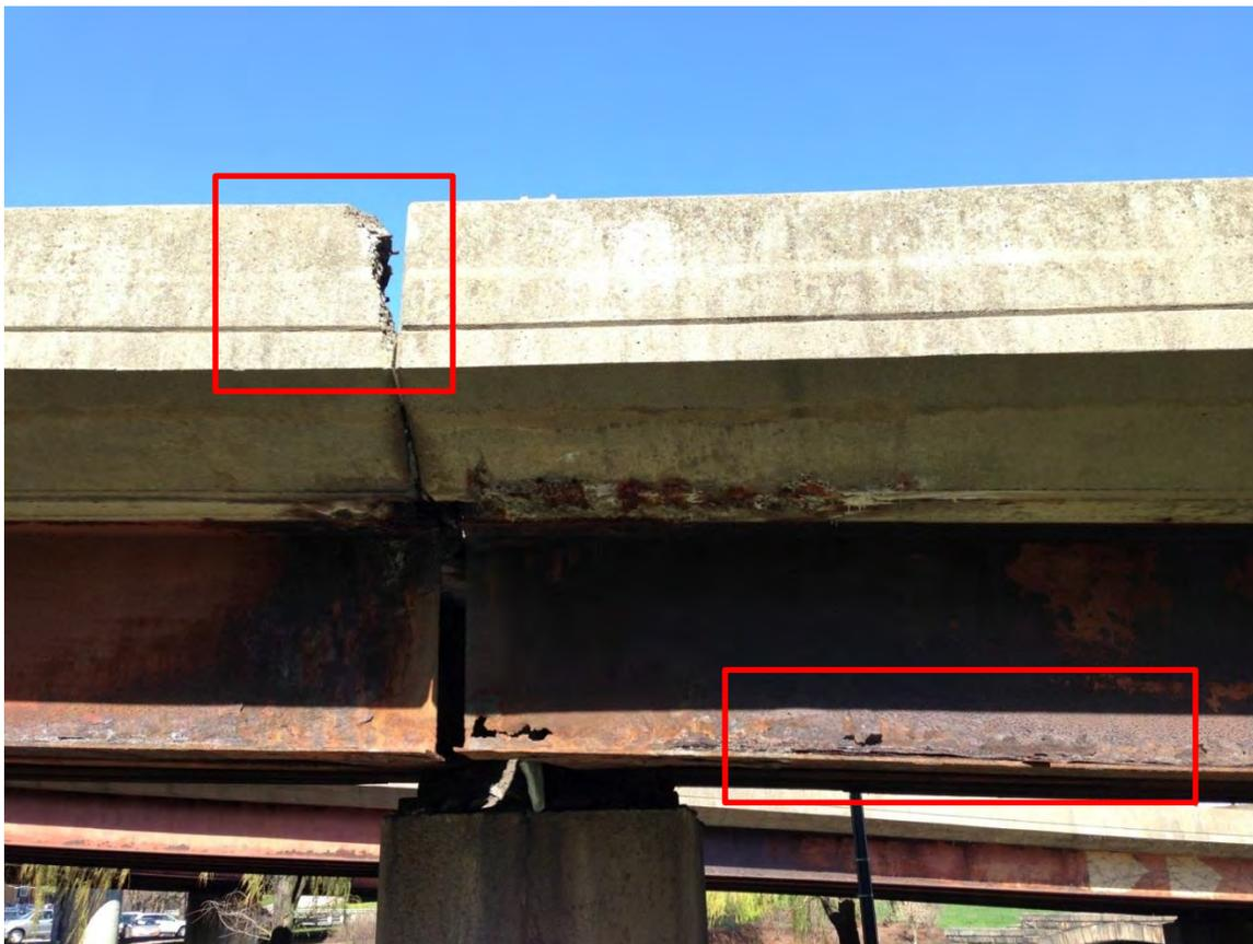
Figure E.9: Side view of the joint from the east on Bridge 4FJ with concrete spalling, delamination, etc.
