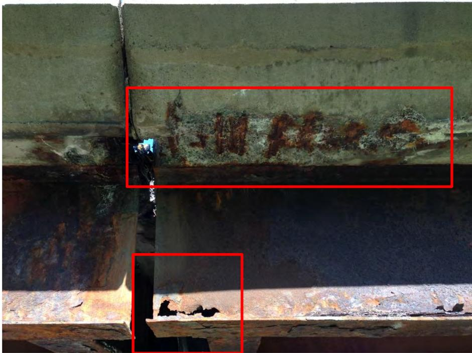
Figure E.10: Section loss, concrete spalling and exposed reinforcement from the exterior view of the joint of Bridge 4FJ.
