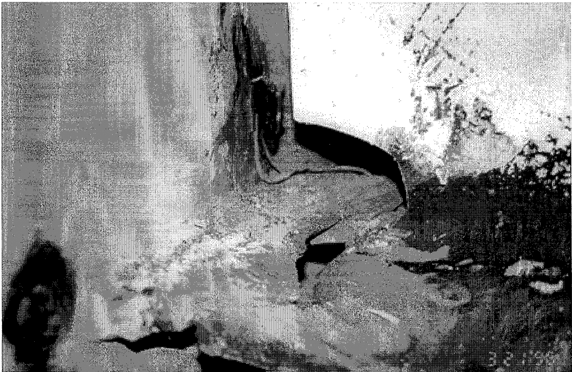
Figure 5.78: Rupture of Bottom Girder Flange (West Girder of Specimen 3)
