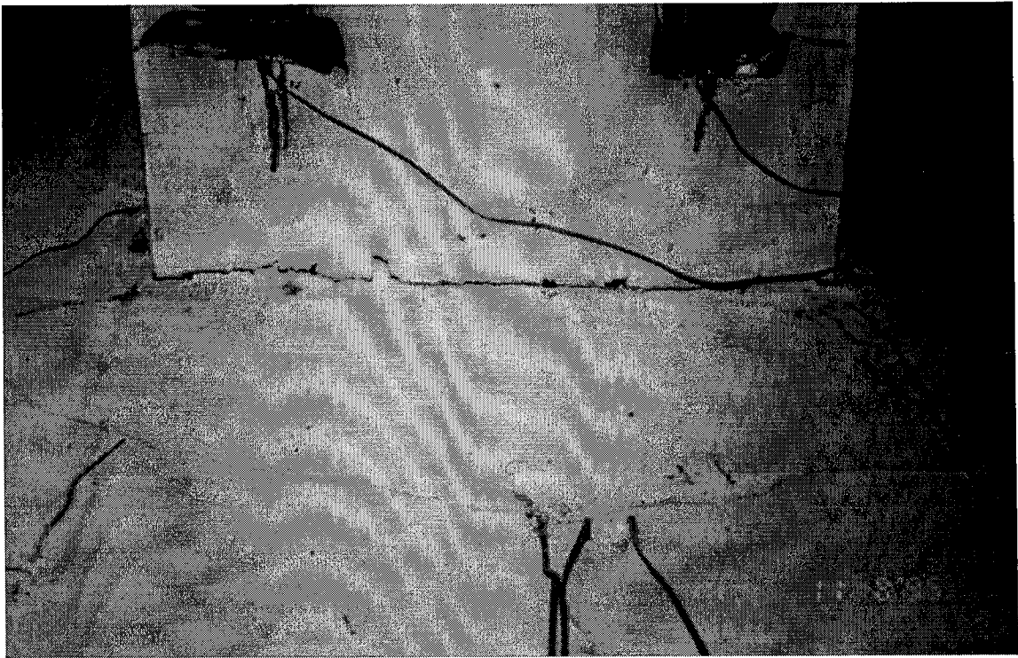
Figure 5.48: Top View of Concrete Slab-Column Interface (West Girder of Specimen 2)
