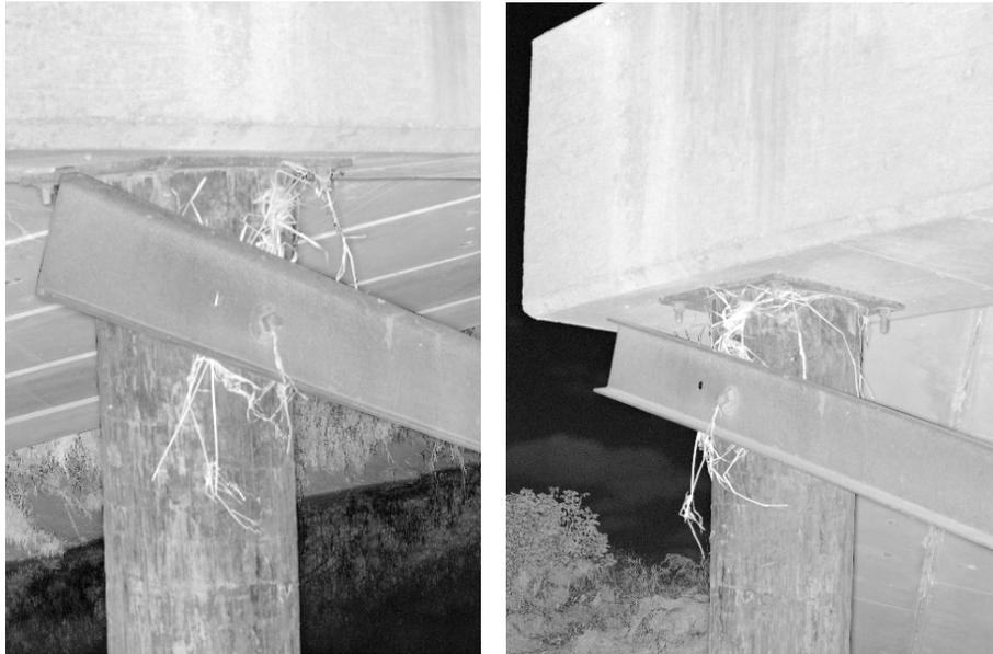
Figure 3.5: Section of testbed bridge point cloud showing grass located between a pier and a brace.
