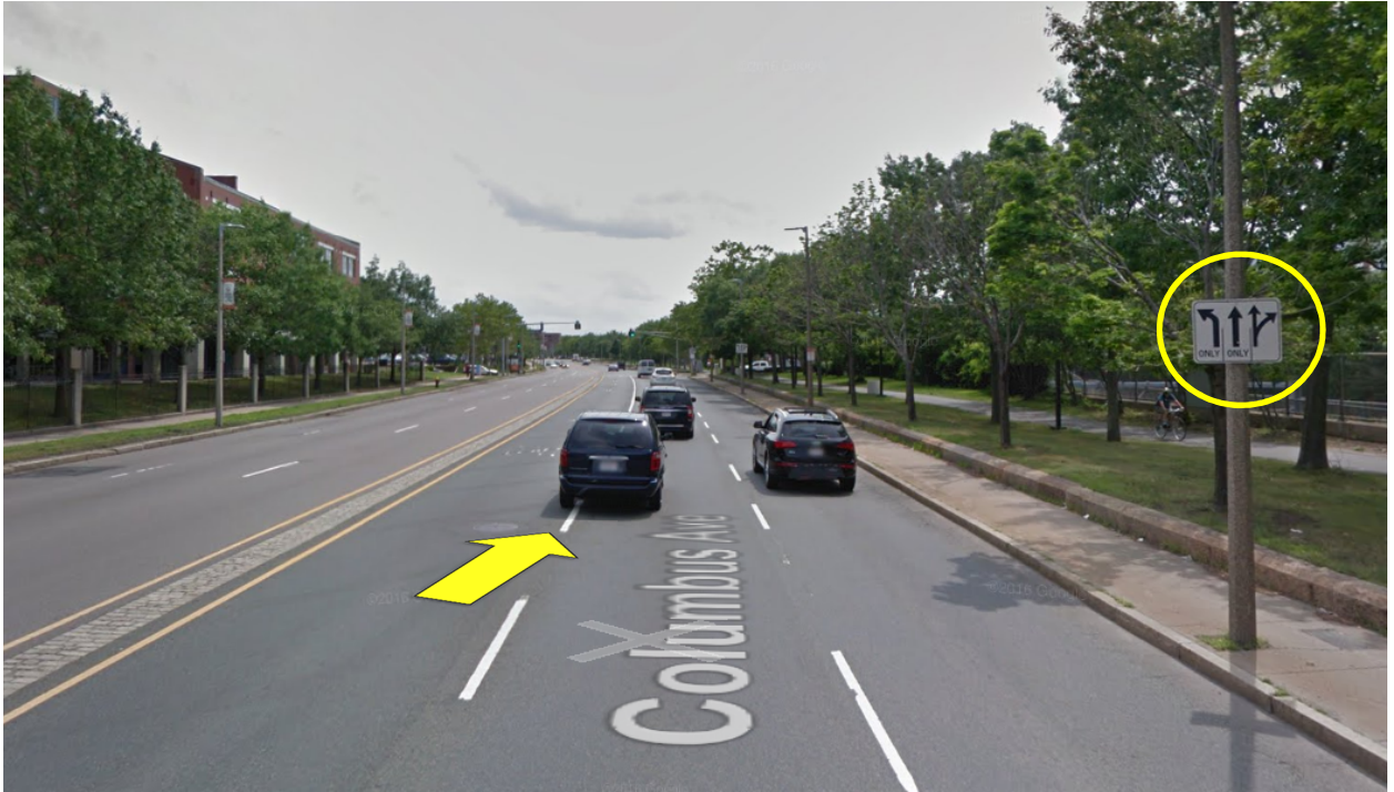
Figure 10: Through Lanes on Columbus Avenue Suddenly Become Turn Lanes, Forcing Drivers to Merge Unexpectedly
