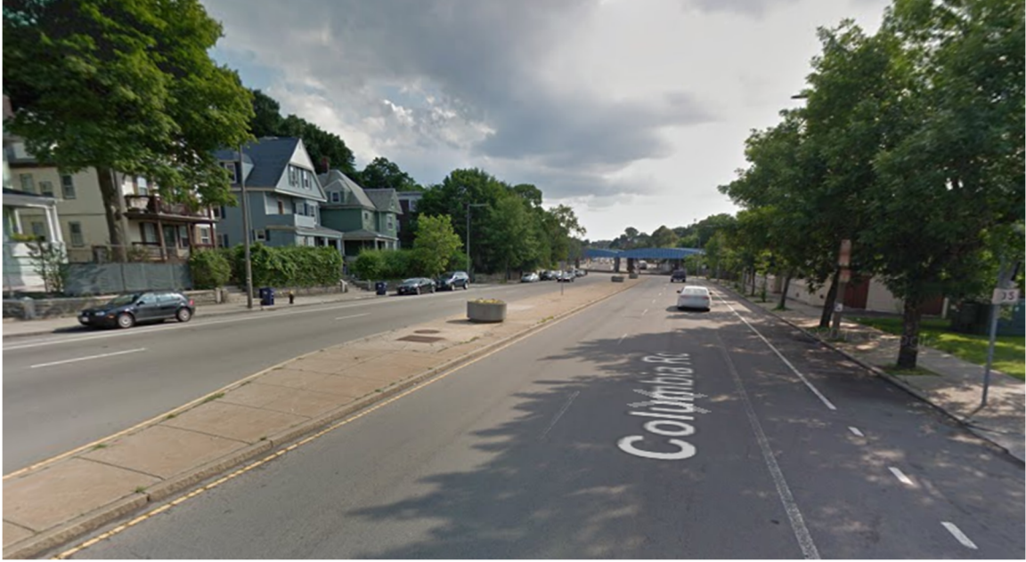
Figure 20: Columbia Road, Boston, an Urban Minor Arterial
