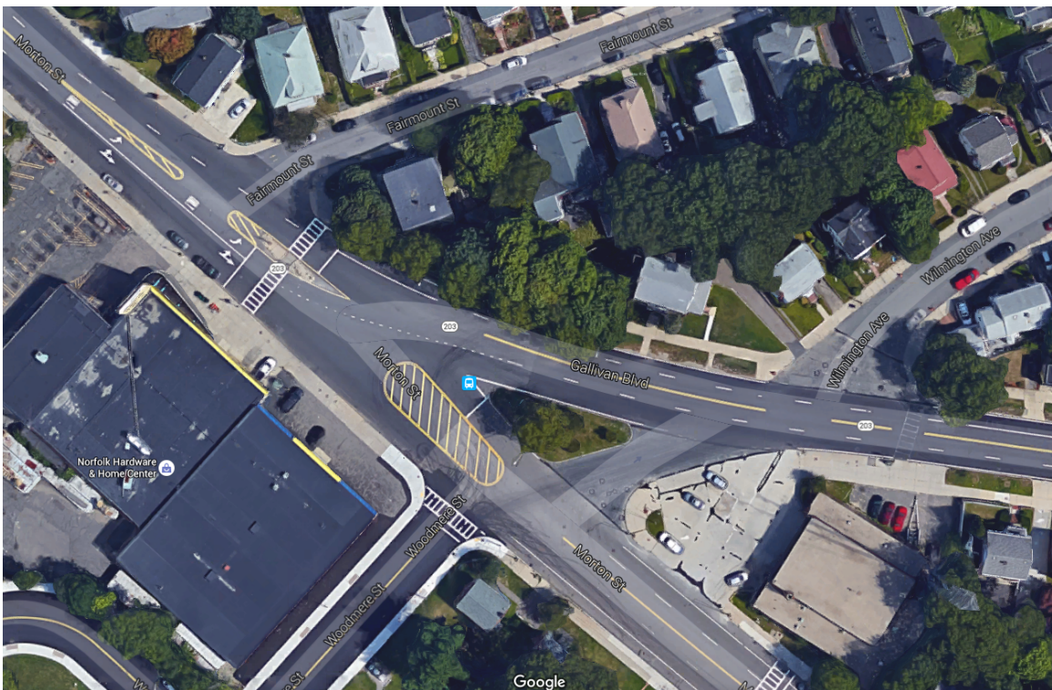
Figure 36: A Candidate for Conversion to a Roundabout: Gallivan Boulevard at Morton Street, Boston
