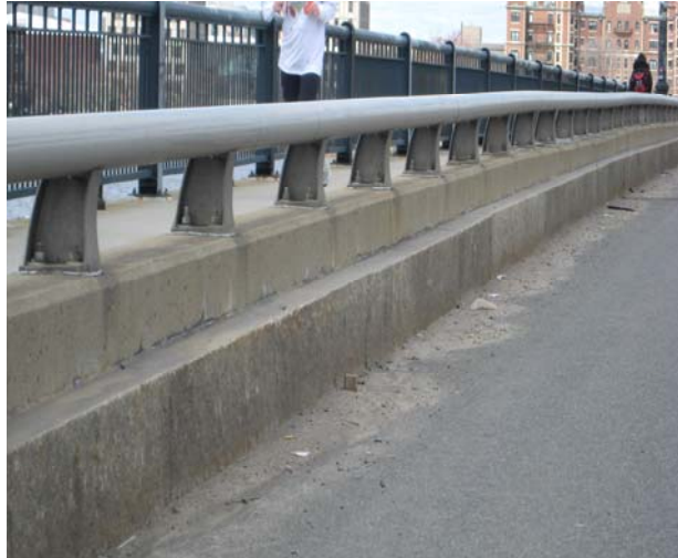
Figure 6.11 – Massachusetts Avenue pedestrian barrier
